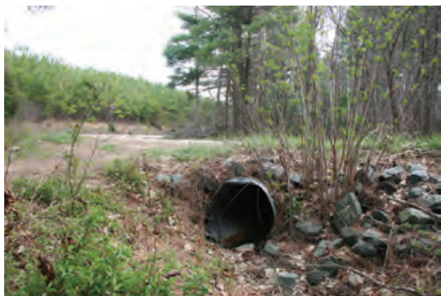
Proper culverts or stream crossings protect water quality during logging operations
