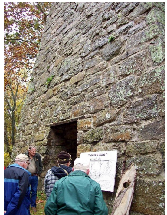
Hardwood charcoal was used to fuel iron furnaces. It is estimated that it took an acre of wood (in the form of charcoal) every day to keep a furnace operating. Photo by: Jennifer Gagnon, Virginia Tech.
